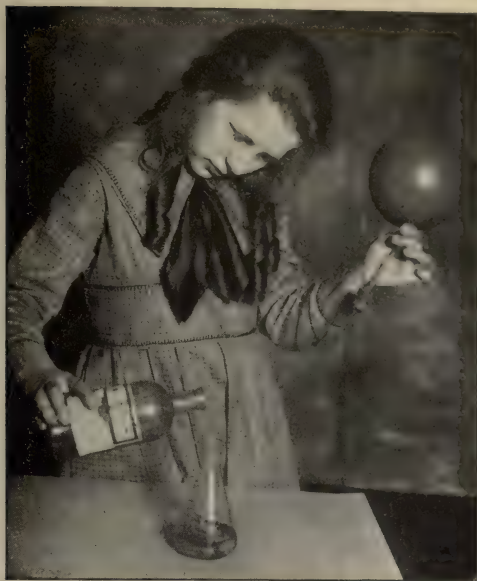
FIG. 163. Adding more acid without losing the gas.
